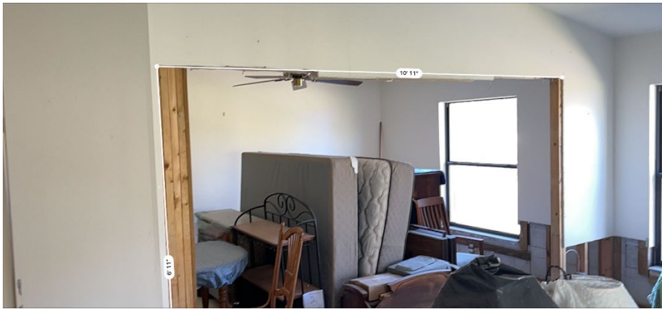
Den wall to be framed and drywalled
