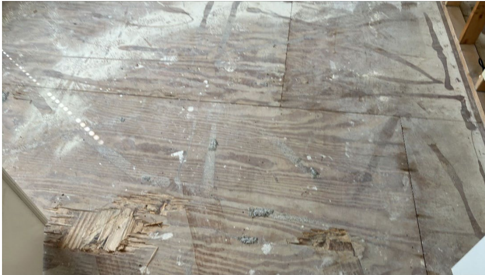
Guest bedroom, subfloor
