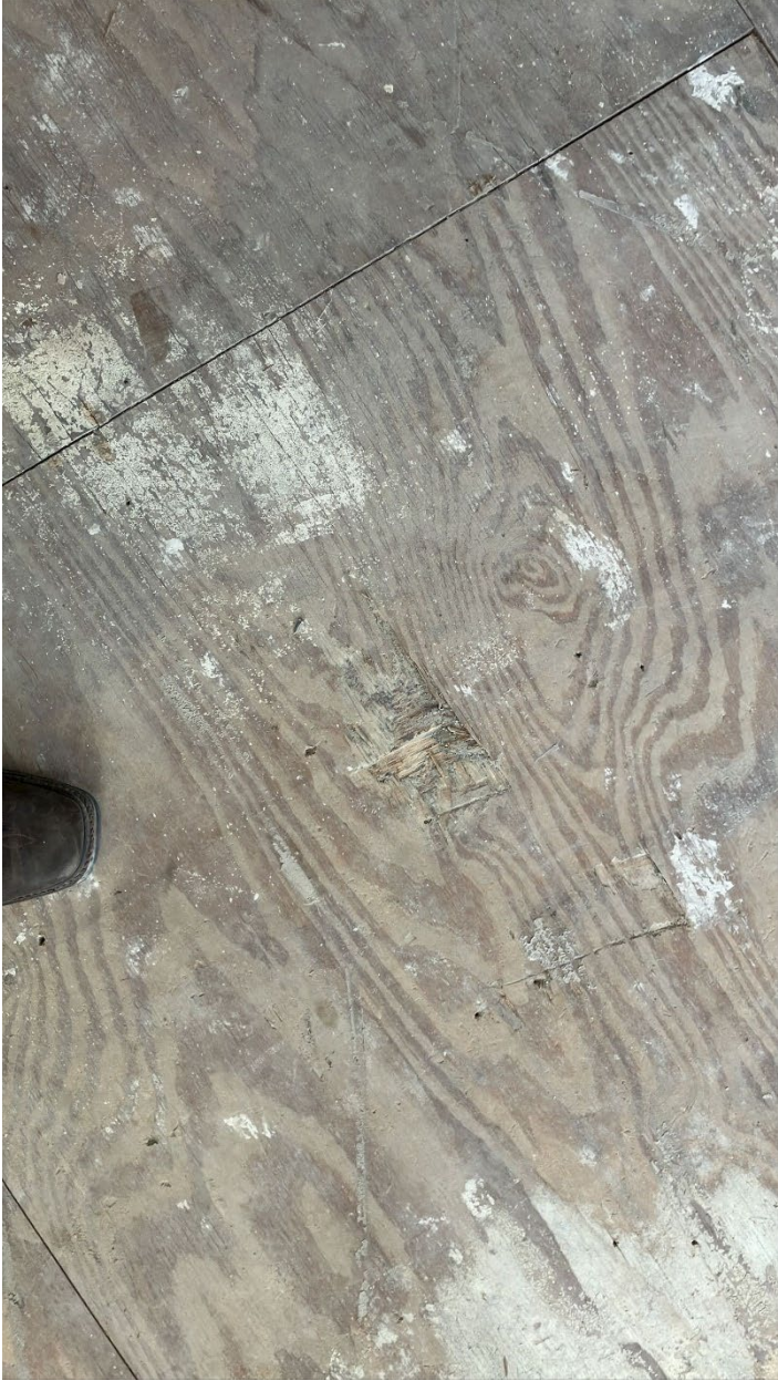
Chipped up sub-floor
