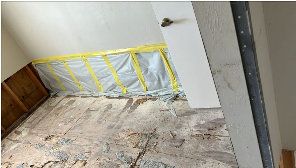
Subfloors guest bedroom two
