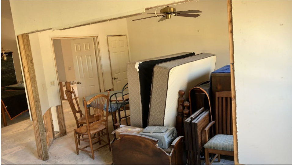
Den wall to be framed and drywalled
