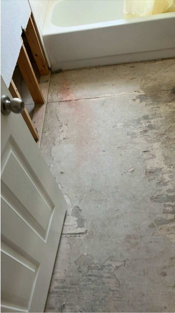
Guest bathroom floor
