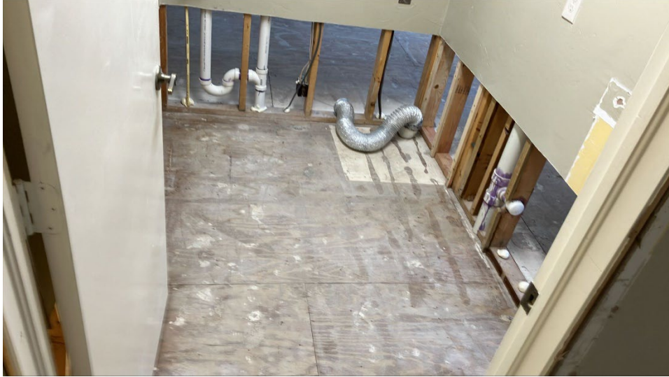
Laundry room subfloor
