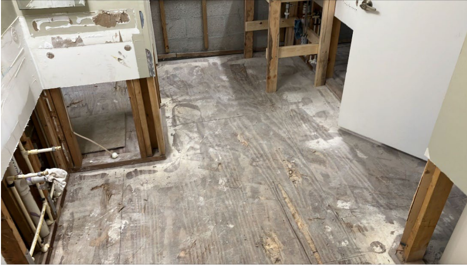
Master bathroom, subfloor
