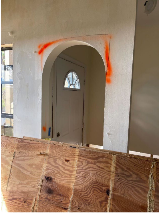
Square off arch in living room
