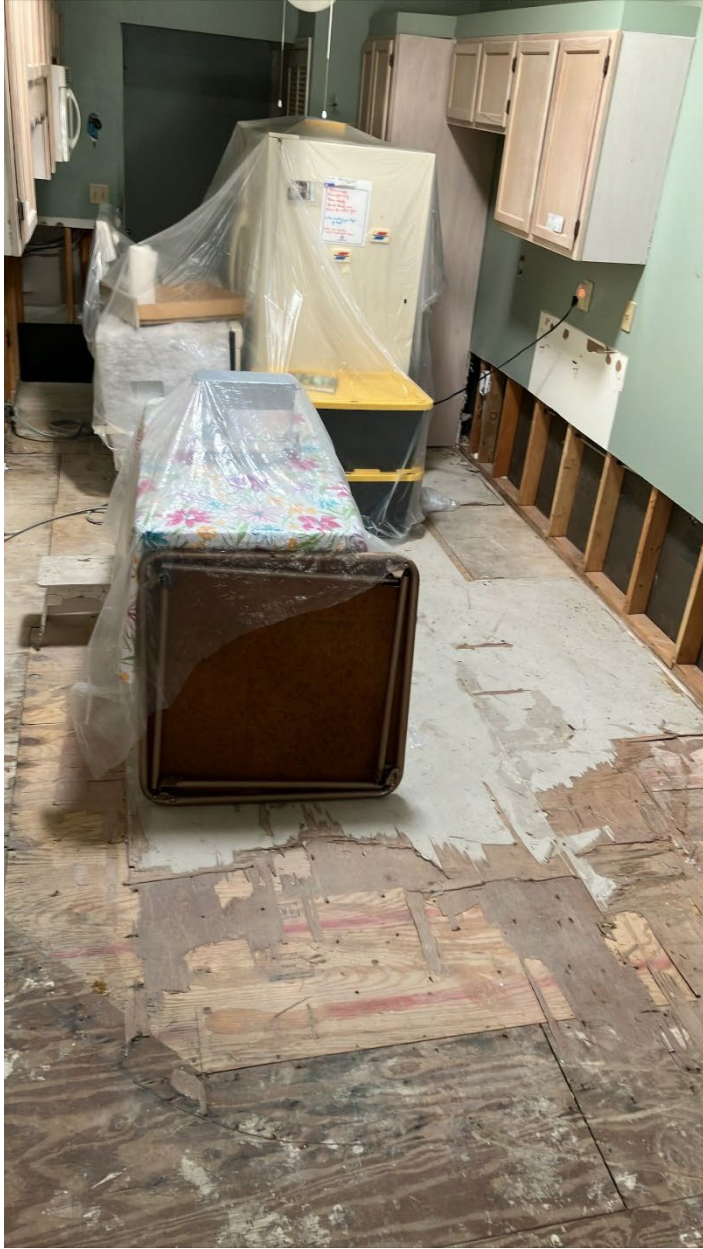
Sub flooring in kitchen
