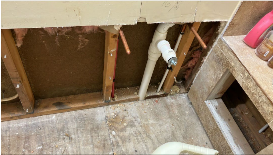
Master bedroom bathroom
