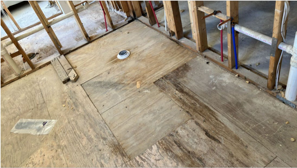
Master bedroom bathroom
