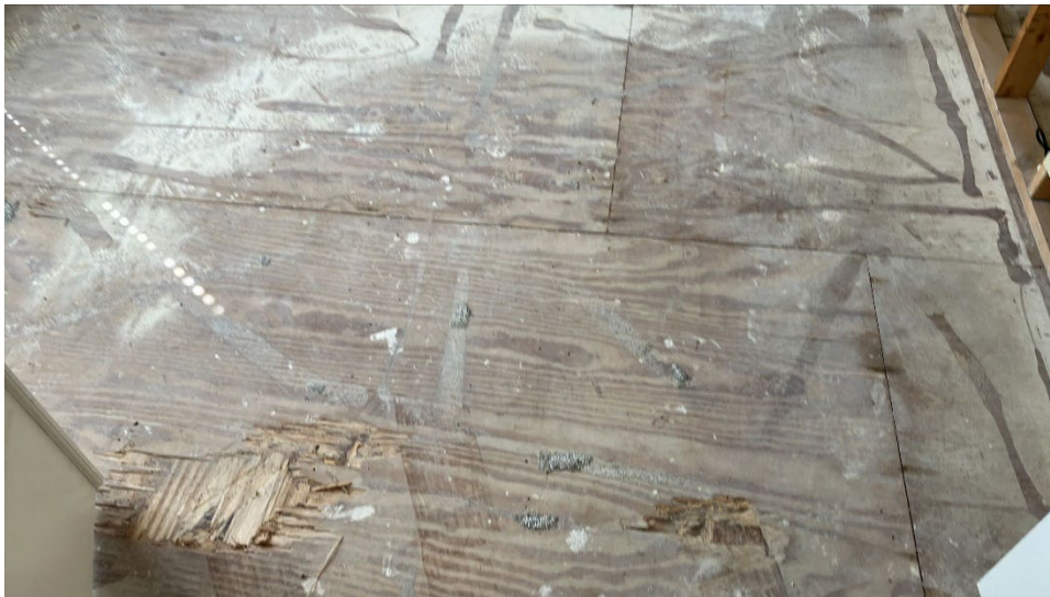
Guest bedroom, subfloor
