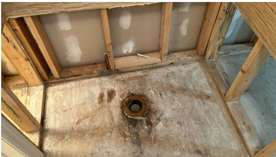
Master bedroom bathroom
