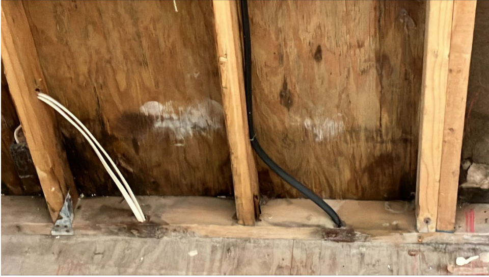
Water damage on plywood exterior in kitchen area
