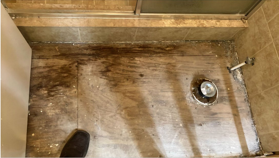
Master bedroom, shower area
