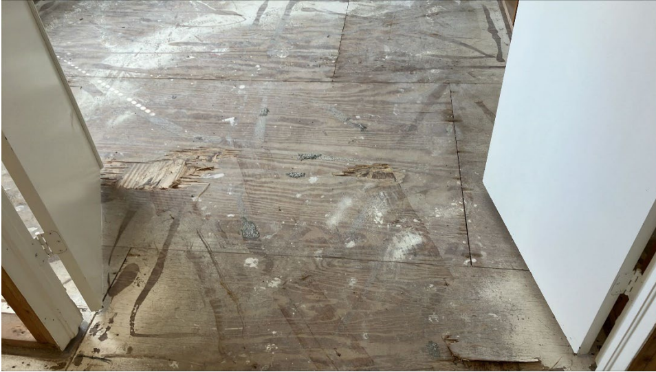
Entrance guest room one
