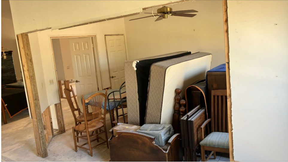
Den wall to be framed and drywalled
