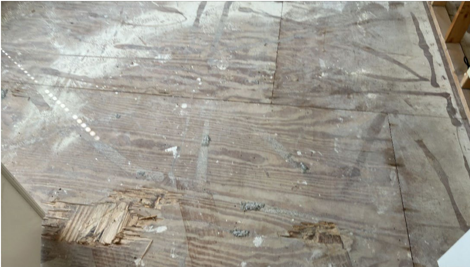
Guest bedroom, subfloor
