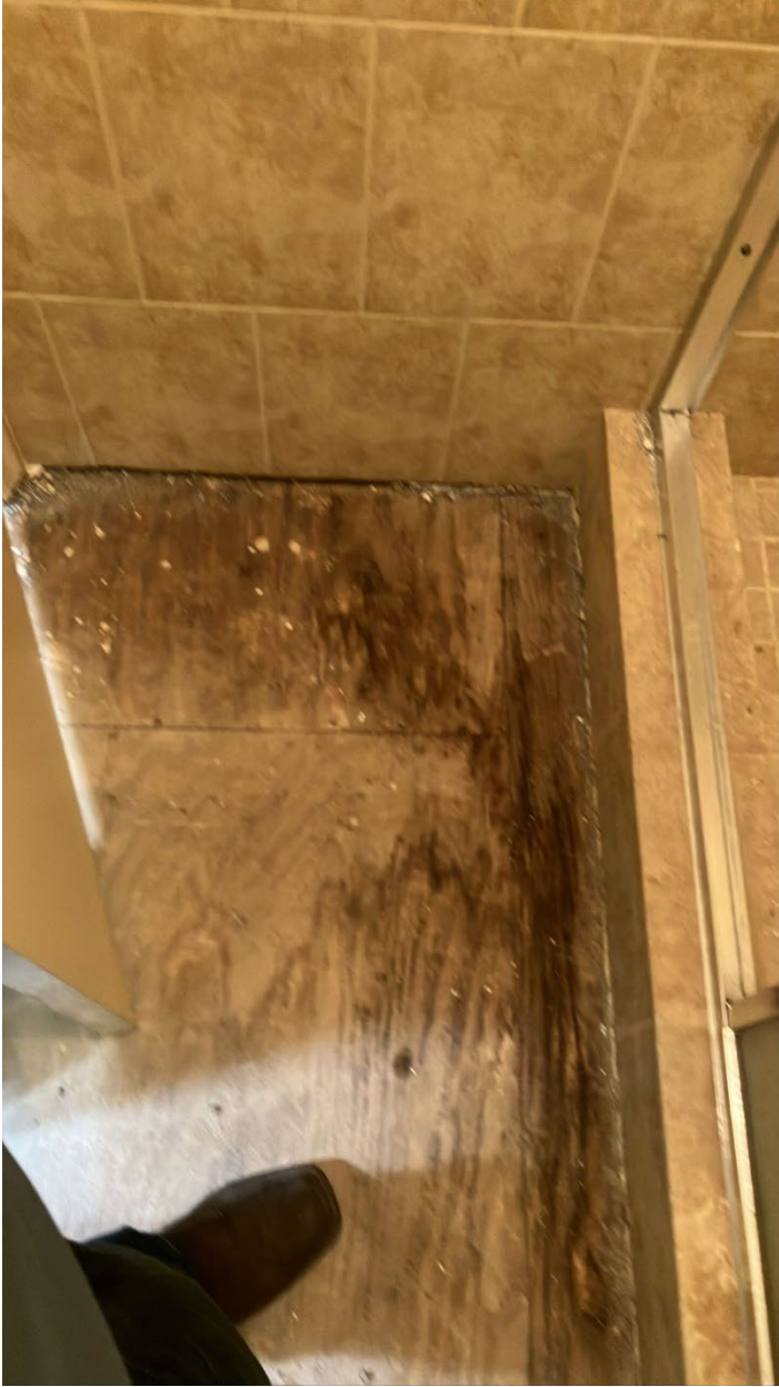
Master bedroom, shower area
