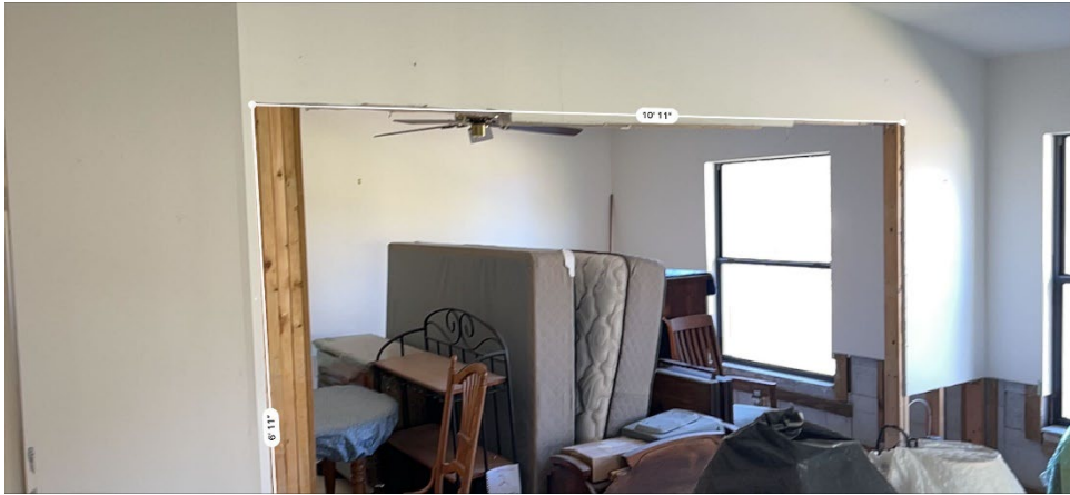
Den wall to be framed and drywalled
