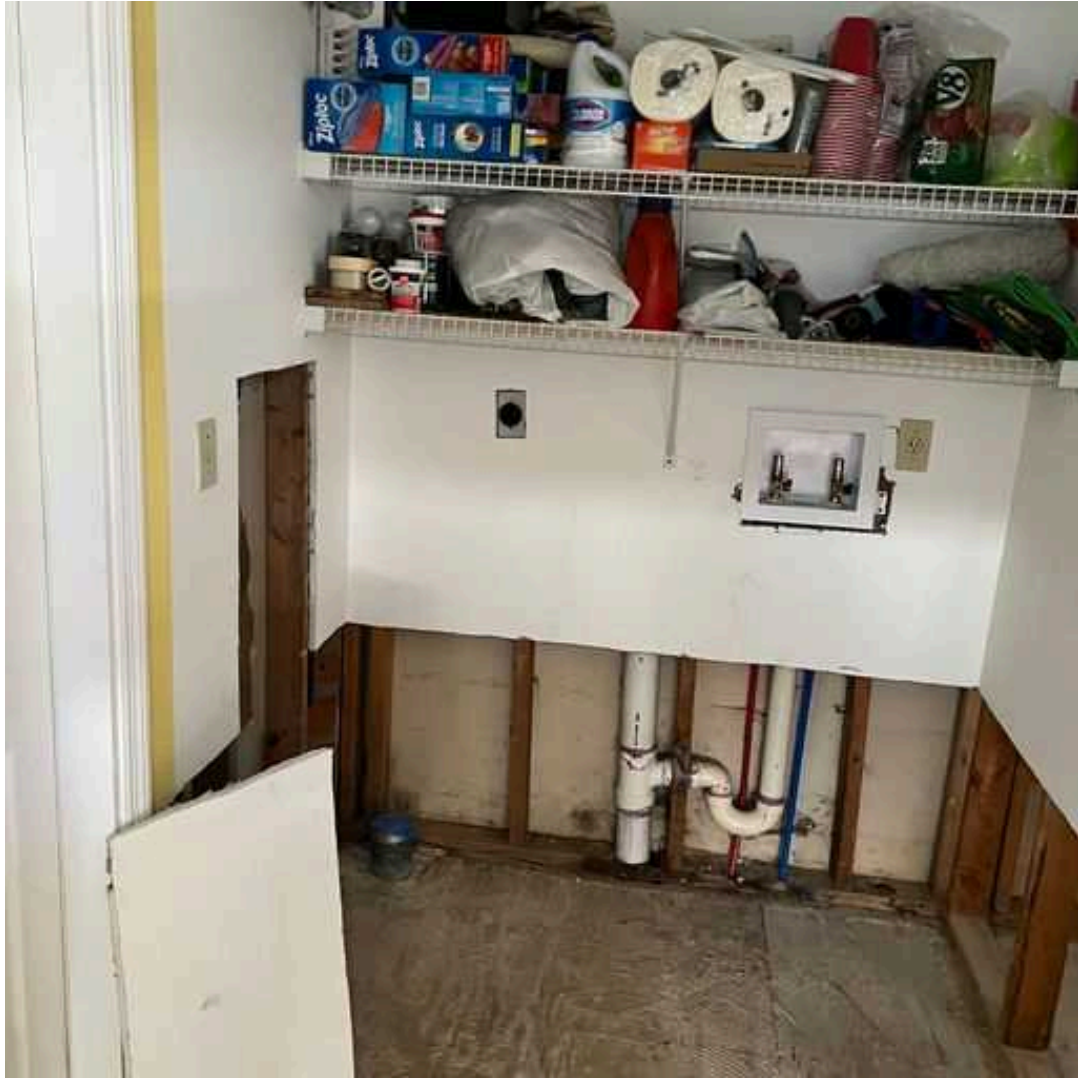
5 Main Level/Laundry Room - 3- Laundry room
