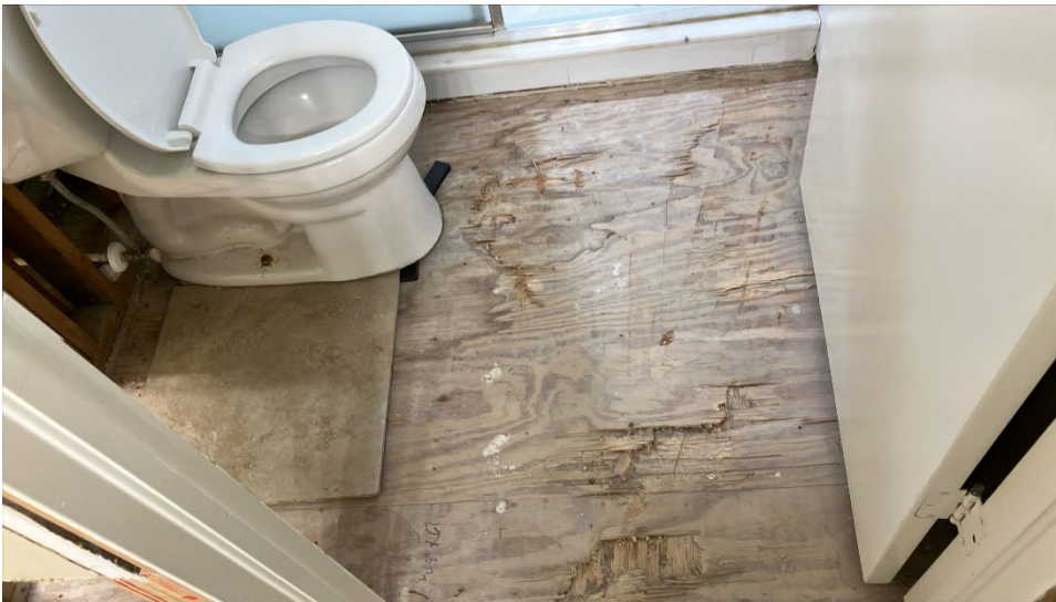
Master bathroom stand up shower area sub for
