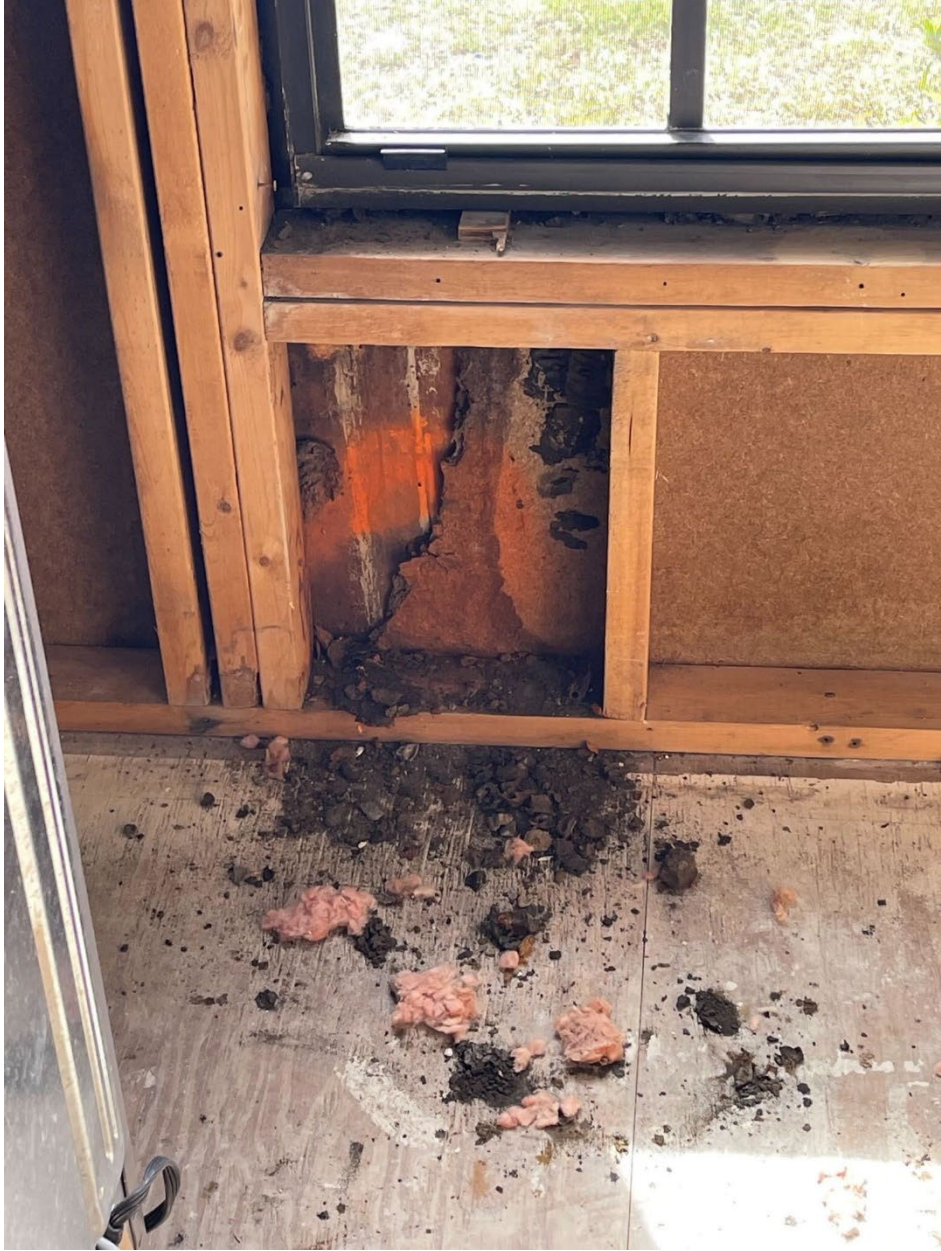
Under living room window, wood sheathing
