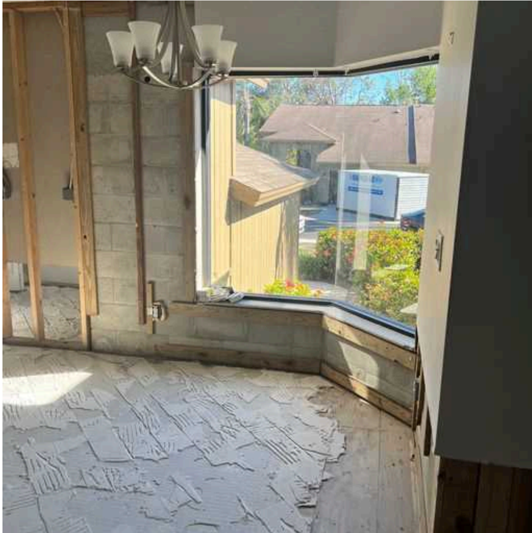
12 Main Level/Dining Room - 1- Dining
