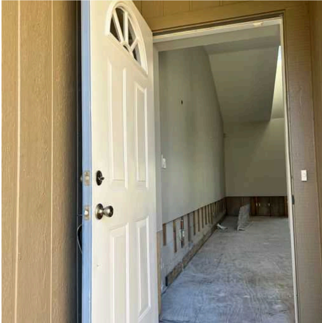
10 Main Level/Entry/Foyer - 2-Entry
