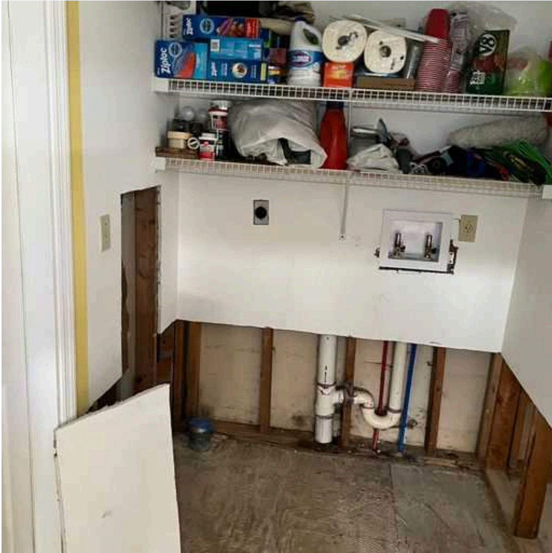
5 Main Level/Laundry Room - 3- Laundry room
